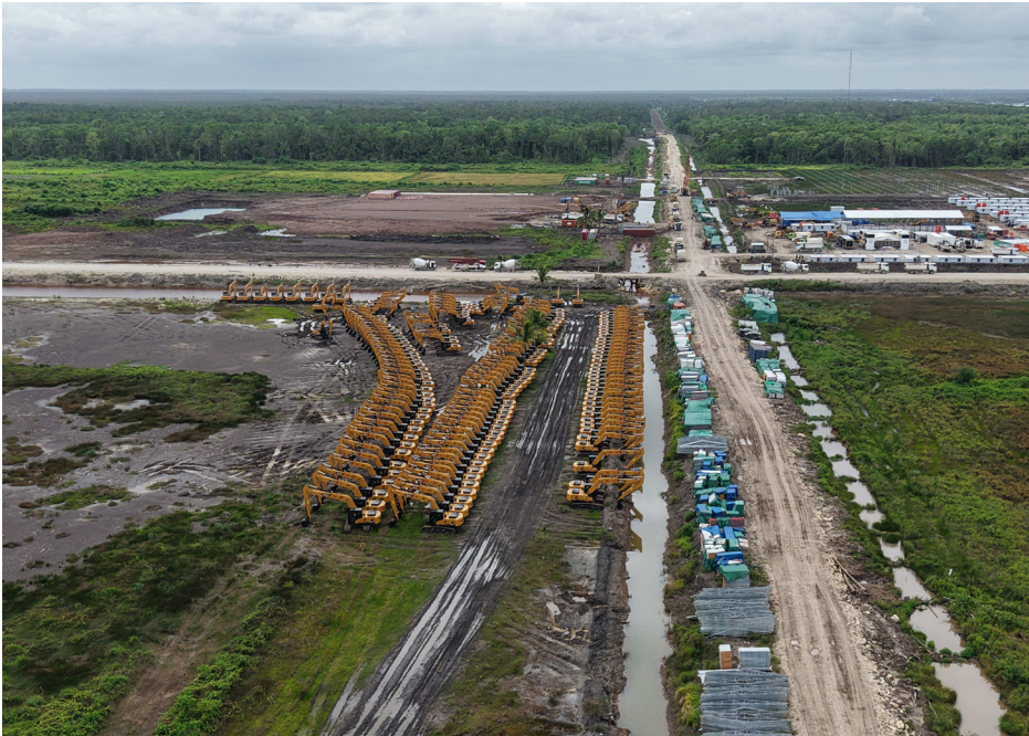
Picture 5. The Johnlin Group basecamp in an area cleared for the 135-km road and rice fields in Wanam. Photo: PUSAKA Bentala Rakyat
